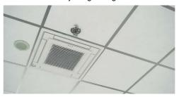
• 2-, 3-, and 4-way airflow patterns are available, enabling installation in the corner of a room.
